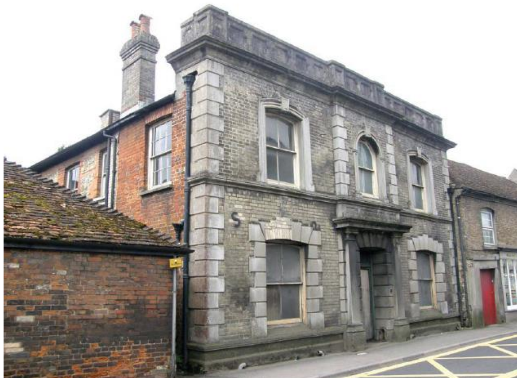
Elevation facing Silver Street
